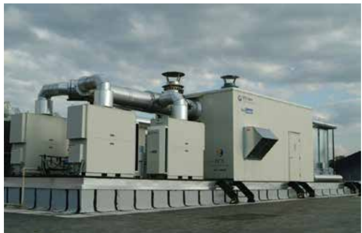
A PureComfort® solution featuring four 60kW Capstone microturbines provide cooling, heating, and power for this supermarket in New York State.
