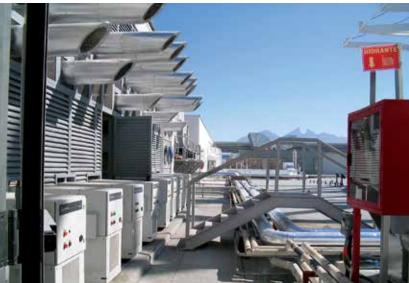
Twenty Capstone C65 microturbines produce 40 percent of the electrical power needed to operate a department store in Monterrey, Mexico.
