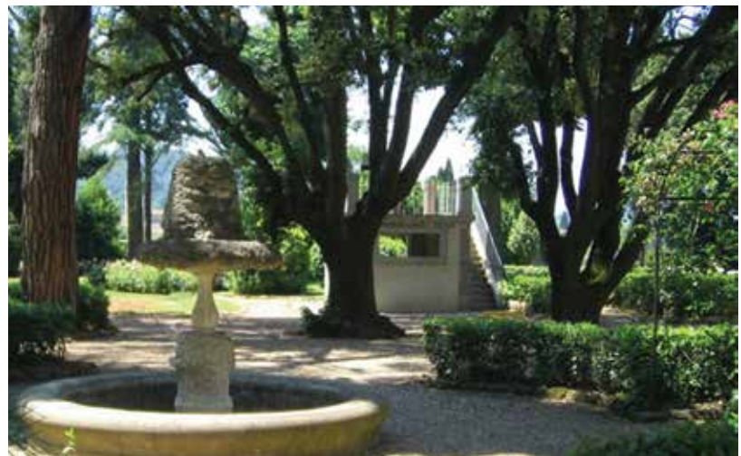
Three Capstone C60 microturbines generate cooling, heating, and power for Villa Olmi Resort in Florence, Italy.
