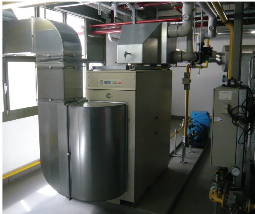
The Capstone C65 cogeneration system saves the hospital €22,500 annually in energy costs.
