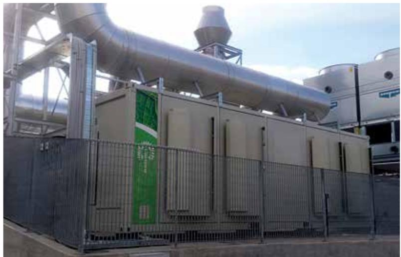
A 365kW ammonia absorption chiller produces chilled water to both refrigerate the warehouse and provide air conditioning to the adjacent offices. Any excess electricity produced can easily be fed into the grid and sold through the national utility system.
