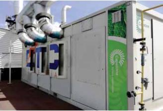
A natural gas-fueled C600 Microturbine reduces fuel and energy costs for the manufacturing plant.
