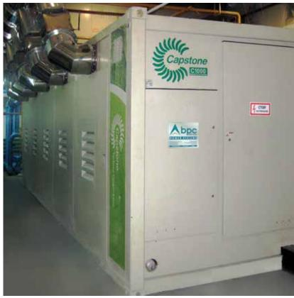
Yakutcement, the local cement and crushed stone manufacturing business, installed two Capstone C1000 Power Packages in a highly efficient CHP application.
